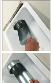
As you initialize the guiding of the duct pipe through the port, put the guide tool through the back of the oval and slide the box up and into the drywall cutout until you have some of the front of the duct protruding through the oval and the back of the duct resting against the guide.
