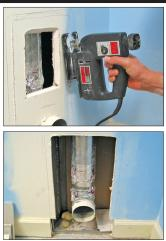
Cut out your hand drawn cut-line on the drywall and cut the original trace line over the baseboard. This will allow the Retro-Fit box to be installed against the drywall. Note the notch in the lower left picture.
