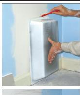
No template is included, so you may want to trace the outer edges of the Retro-Fit box and then by-hand, transfer an imaginary line about 7/8" in from that on the two sides and **about 3/8" on the top.** If you can hold it off the floor about 3/8" it will assist with the installation But not too much, as we later. hope to caulk the gap at the bottom or have the future flooring material cover it.
