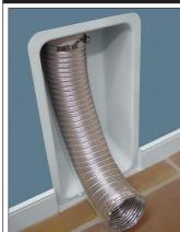
Once you get the pipe through the top port, work the Retro-Fit box up and against the drywall. Use two threaded screws to secure the bottom of the Retro-Fit box to the bottom plate. Fastening the bottom to the bottom plate is actually all the affixing you will need as the Snaplock pipe holds the top of the box firmly against the drywall. De-burr the Snaplock pipe and attach approved flexible duct. Caulk and touchup the baseboard. Put your tools away and grab a beer.
