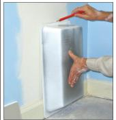
No template is included, so you may want to trace the outer edges of the Retro-Fit box and then by-hand, transfer an imaginary line about 7/8" in from that on the two sides and about 3/8" on the top. If you can hold it off the floor about 3/8" it will assist with the installation But not too much, as we later. hope to caulk the gap at the bottom or have the future flooring material cover it.
