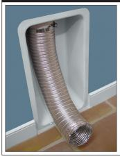
Once you get the pipe through the top port, work the Retro-Fit box up and against the drywall. Use two threaded screws to secure the bottom of the Retro-Fit box to the bottom plate. Fastening the bottom to the bottom plate is actually all the affixing you will need as the Snaplock pipe holds the top of the box firmly against the drywall. De-burr the Snaplock pipe and attach approved flexible duct. Caulk and touchup the baseboard. Put your tools away and grab a beer.
