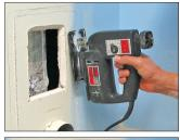
Cut out your hand drawn cut-line on the drywall and cut the original trace line over the baseboard. This will allow the Retro-Fit box to be installed against the drywall. Note the notch in the lower left picture.
