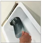
As you initialize the guiding of the duct pipe through the port, put the guide tool through the back of the oval and slide the box up and into the drywall cutout until you have some of the front of the duct protruding through the oval and the back of the duct resting against the guide.
